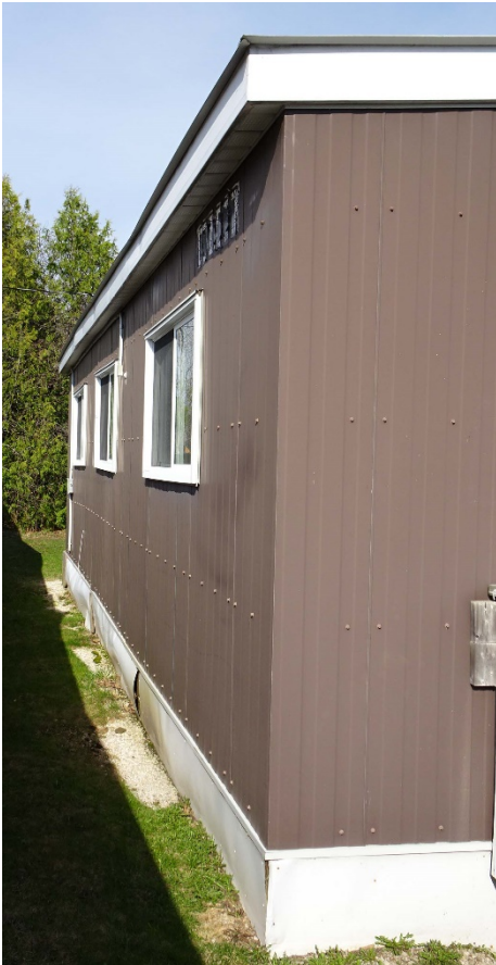
DEPOT BUILDING – SOUTH-EAST VIEW
