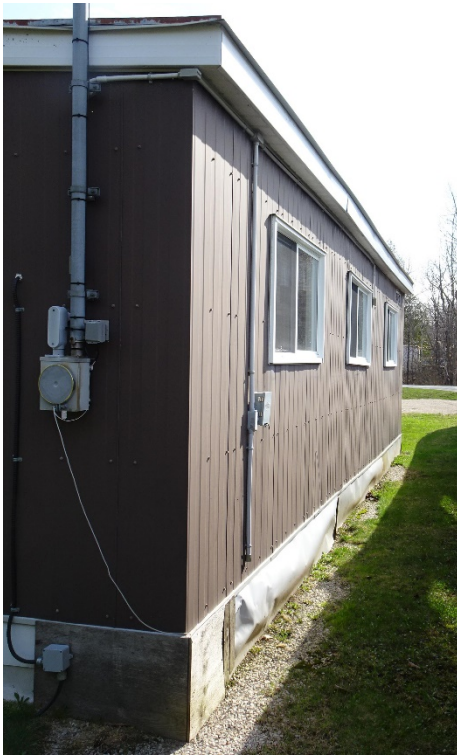
DEPOT BUILDING – SOUTH-WEST VIEW
